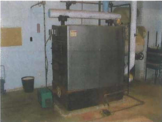
Mechanical Picture #5 Hot water heating boiler
