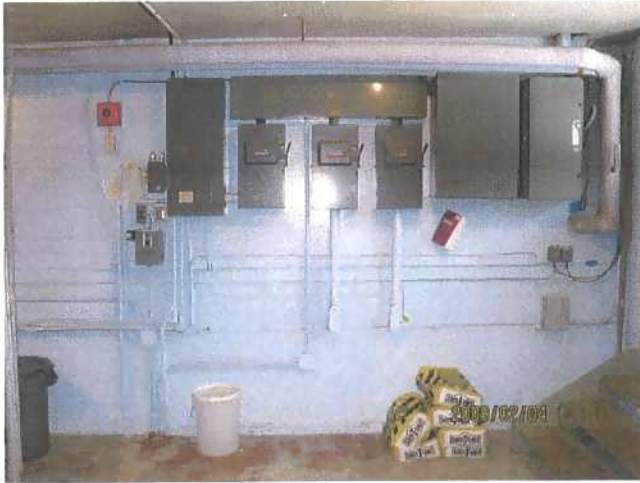
Electrical Picture #1 Electrical Service Entrance Equipment in Boiler Room.
