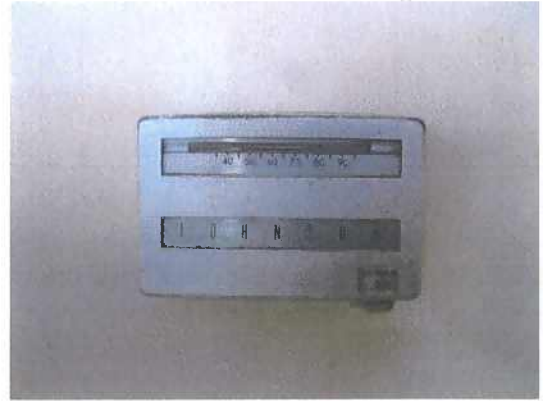
Mechanical Picture #12 Original pneumatic thermostat
