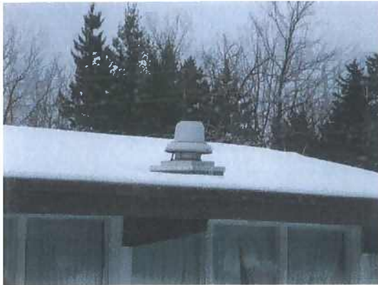
Mechanical Picture #11 Typical roof top exhaust fan.
