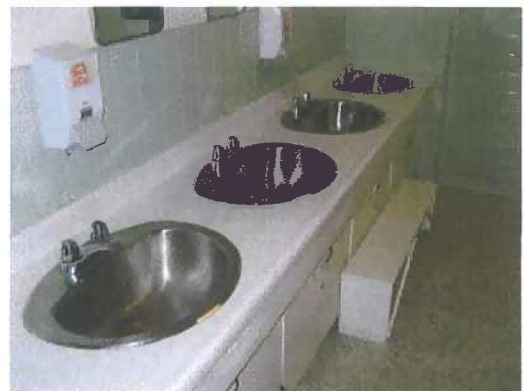
Mechanical Picture #2 Lavatories stained from dripping faucets
