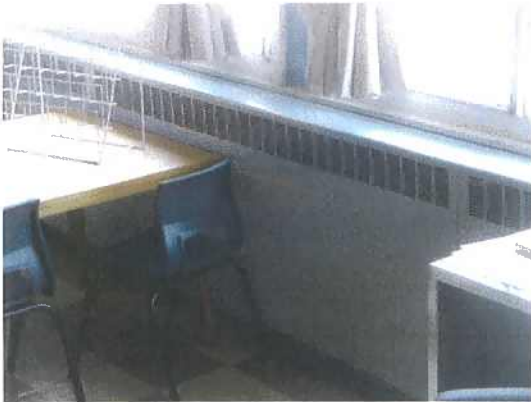
Mechanical Picture #9 Typical wall fin radiation
