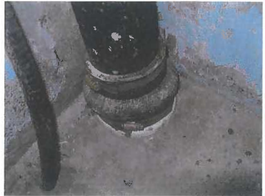
Mechanical Picture #4 Repaired rain water leader
