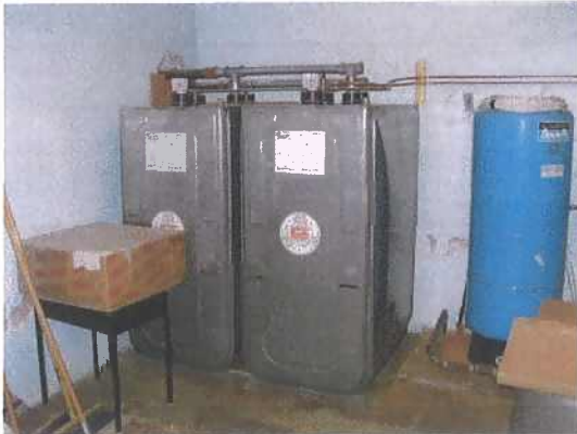
Mechanical Picture #7 Furnace oil tanks
