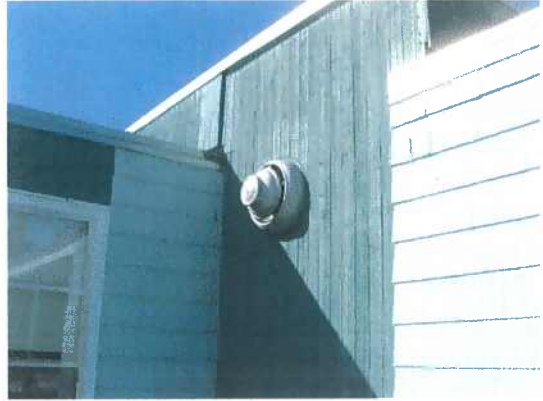
Mechanical Picture #12 Wall exhaust fan
