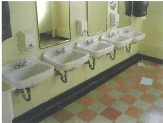
Mechanical Picture #1 Existing lavatories
