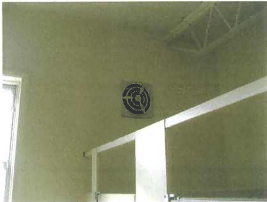
Mechanical Picture #13 Wall exhauster (washrooms)
