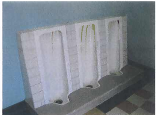
Mechanical Picture #2 Existing urinals
