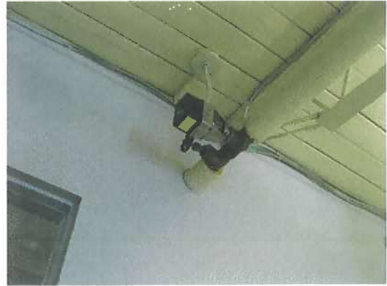
Mechanical Picture #14 Zone valve (one per two classrooms)
