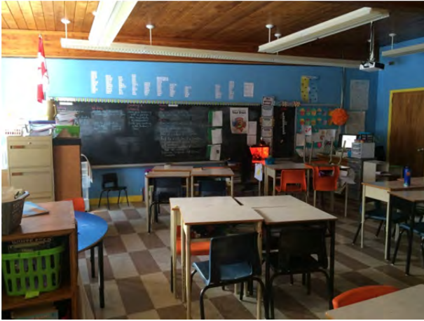
Photo 4.8.1 – Typical classroom finishes. Linoleum tile floor, painted walls, wood finished ceiling.
