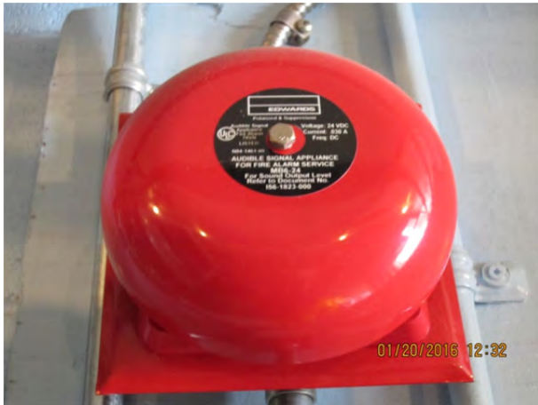
Photo 4.5.25 – Typical fire alarm bell
