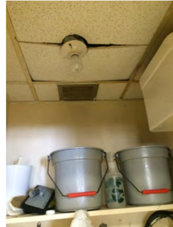
Photo 4.4.8 – Typical exhaust grill for exhaust fans
