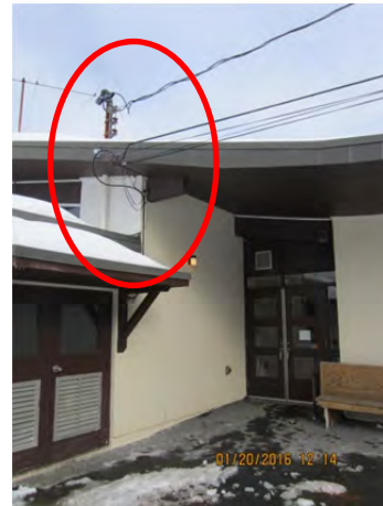
Photo 4.5.2 – Overhead power lines for school service into boiler room
