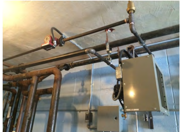
Photo 4.4.4 – Mechanical room unit heater
