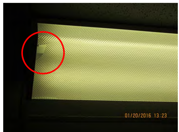
Photo 4.5.30 – Crack in lens of 1'x4' fluorescent luminaire in the boys washroom
