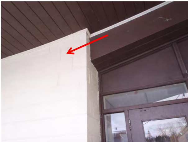
Photo 4.1.3 – Step crack in block mortar on southeast side
