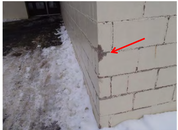
Photo 4.1.4 – Exposed grout and area of material loss. Southeast corner of mechanical room
