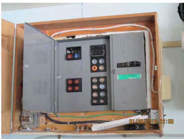
Photo 4.5.5 – 100A, 120/240V, 1-phase main fuse panel located in Portable Classroom
