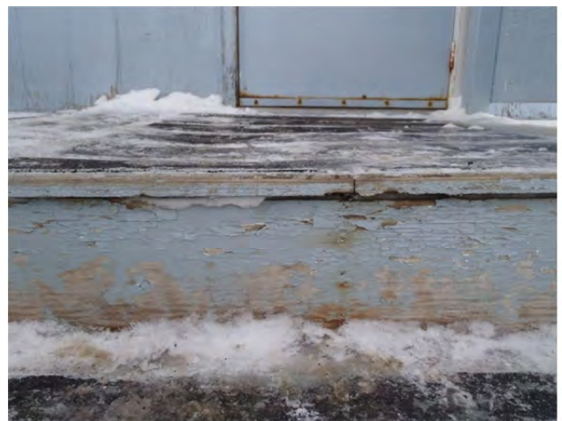
Photo 4.6.6 – Rotted area at top landing of portable classroom stair/ramp
