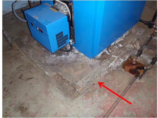
Photo 4.1.8 – Deteriorated housekeeping pad below boiler
