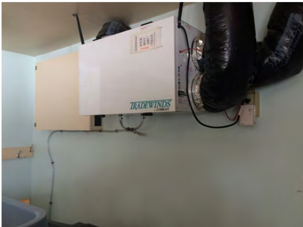
Photo 4.4.9 – Out building heat recovery ventilator (HRV)
