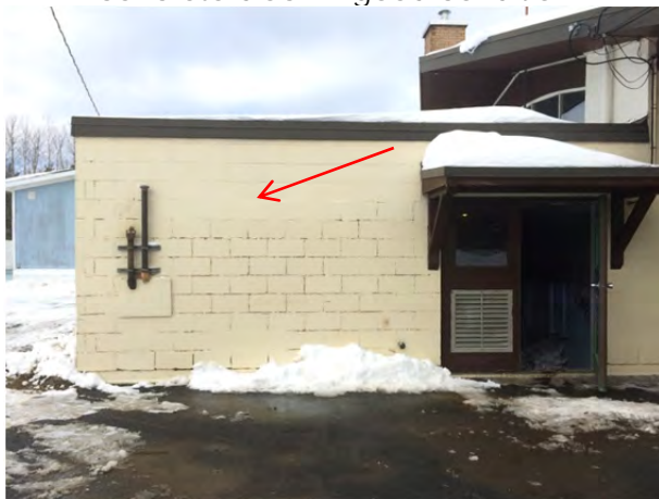
Photo 4.2.11 – North face of boiler room. Located at east side of school. Painted joints in concrete block peeling
