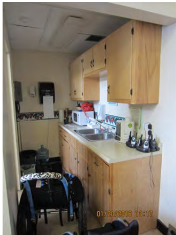
Photo 4.5.15 – Surface-mounted 1'x4' luminaire in the office kitchenette
