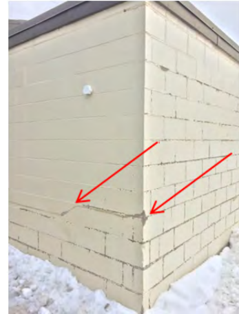
Photo 4.2.14 – South east corner of boiler room. Damages to surface paint and to the concrete block
