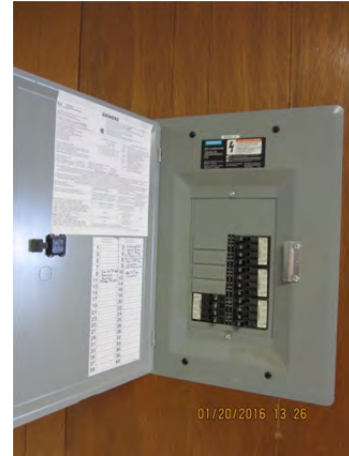
Photo 4.5.8 – 100A, 120/240V, 1-phase, 3-wire Siemens panel
