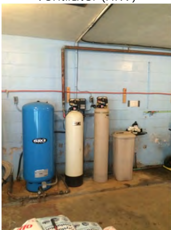
Photo 4.4.11 – Domestic water entrance equipment included pressure tank and water conditioners
