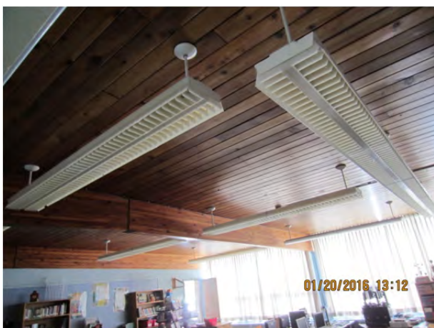
Photo 4.5.11 – Typical suspended 1'x4' fluorescent luminaires in the classrooms
