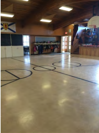
Photo 4.8.7 – Gymnasium finishes. vinyl tile floor, wood panel walls, wood finish ceiling.
