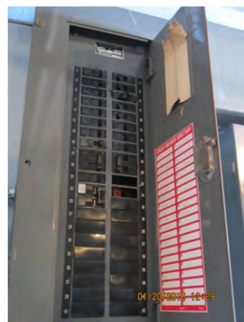
Photo 4.5.6 – 200A, 120/240V, 1-phase, 3-wire panel located in the Boiler Room
