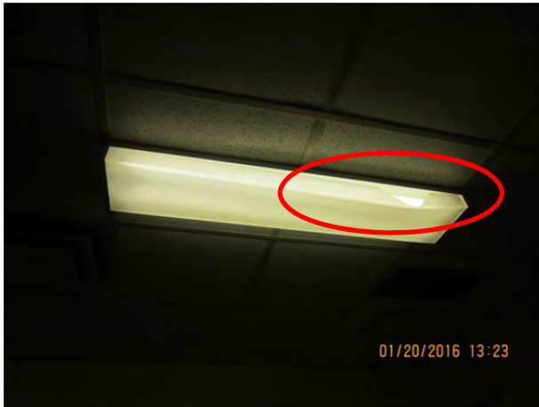
Photo 4.5.31 – Additional cracked lens on 1'x4' surface-mounted fluorescent luminaire in boys washroom
