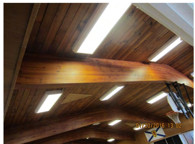
Photo 4.5.12 – 2'x4', 4-lamp fluorescent surface-mounted luminaires in gymnasium
