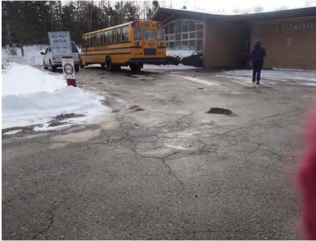
Photo 4.6.1 – Cracking in asphalt on bus loop
