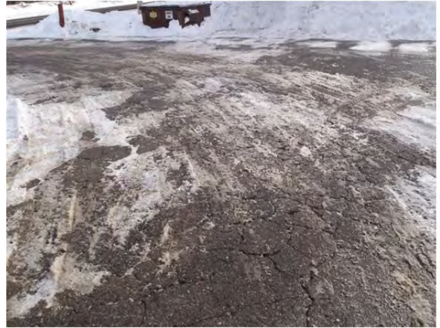
Photo 4.6.2 – Significant cracking in asphalt on bus loop
