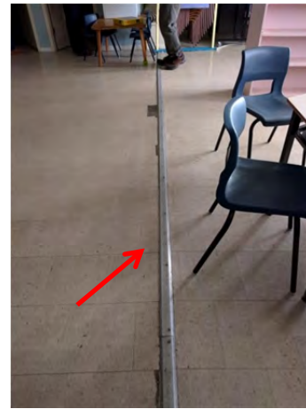
Photo 4.1.10 – High point in classroom portable floor
