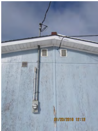
Photo 4.5.3 – Overhead power lines for portable classroom service
