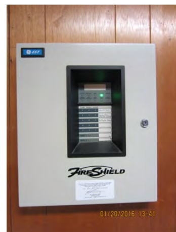
Photo 4.5.24 – GE EST – Fireshield Fire Alarm Control Panel
