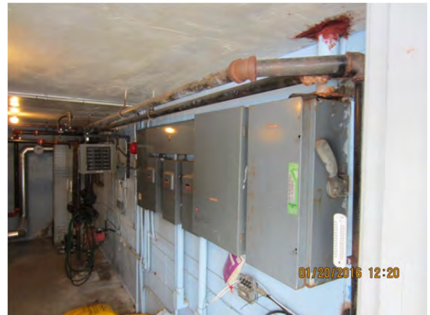
Photo 4.5.4 – Main distribution equipment
