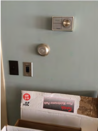
Photo 4.4.7 – Out building Thermostat and humidistat controls
