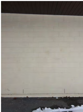
Photo 4.2.9 – East face at north side. Painted concrete block in good condition
