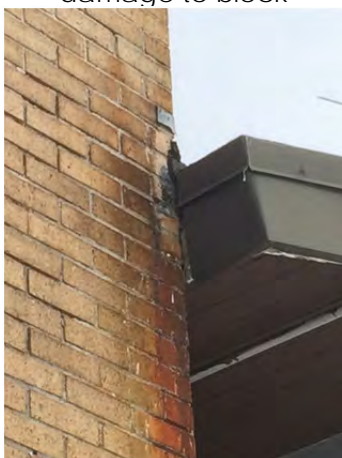
Photo 4.2.17 – Damage at connection between chimney and roof over stage area
