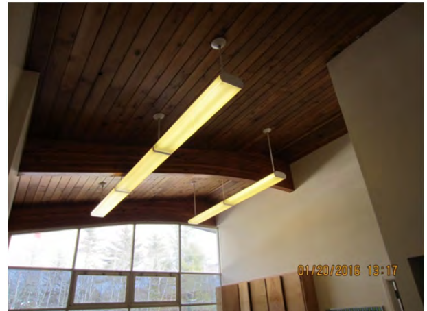
Photo 4.5.14 – Typical 1'x4' suspended fluorescent luminaires in office area
