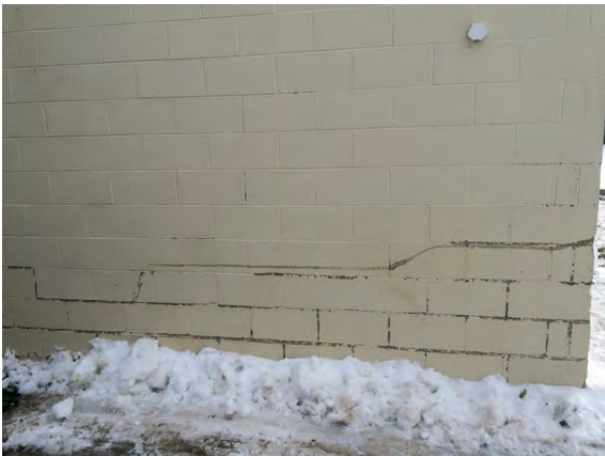
Photo 4.2.15 – South face of boiler room. Paint peeling between concrete block joints and damage to block
