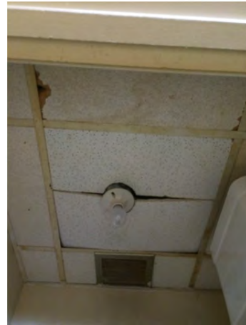
Photo 4.8.4 – Janitor Closet ceiling tile damaged and should be replaced.
