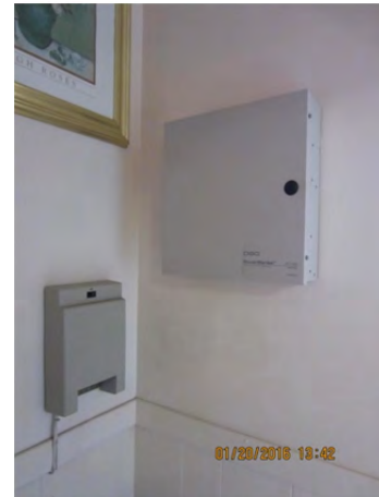
Photo 4.5.26 – Security system control panel
