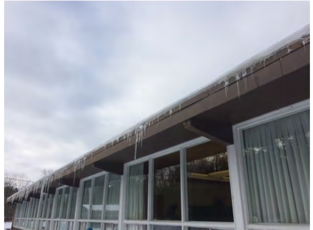
Photo 4.2.2 – North face, roof edge. Underside of roof overhang finished with wood
