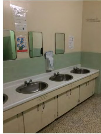
Photo 4.8.2 – Typical washroom finishes, terrazzo floor, tile backsplash at counter, painted walls with suspended ceiling tile.
