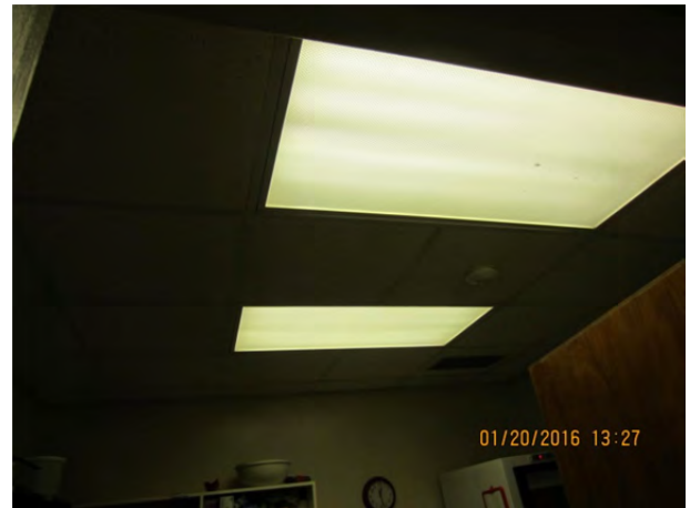
Photo 4.5.16 – Typical 2'x4' recessed fluorescent luminaires in the kitchen
