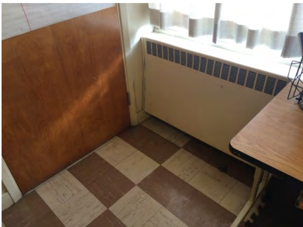
Photo 4.4.5 – Typical hot water baseboard heater
