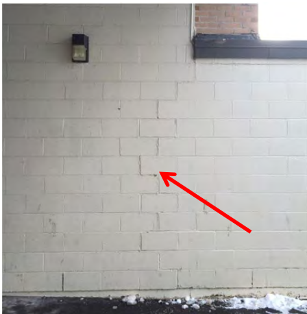
Photo 4.1.5 – Cracks in block mortar at area between the mechanical room and stage
