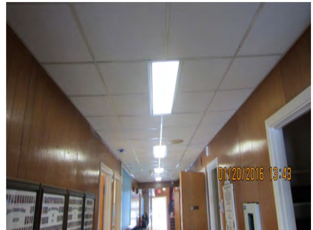
Photo 4.5.10 – Typical 1'x4' recessed fluorescent corridor luminaires
