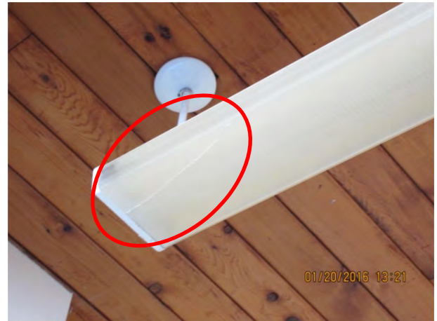
Photo 4.5.32 – Cracked lens of suspended 1'x4' luminaire in Principals office
