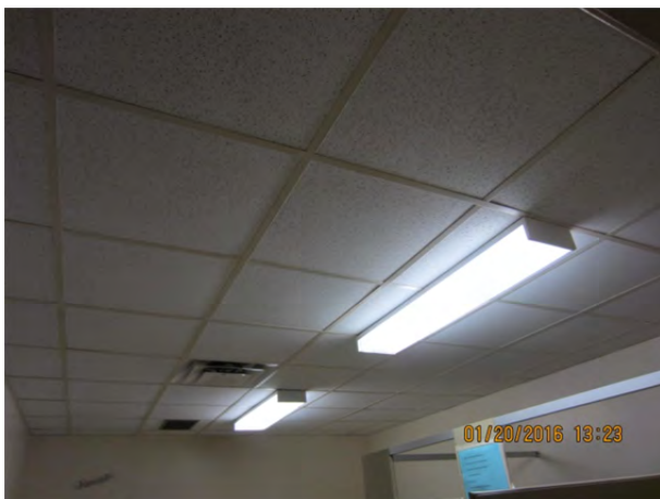
Photo 4.5.17 – Typical surface-mounted 1'x4' fluorescent luminaires in the washrooms
