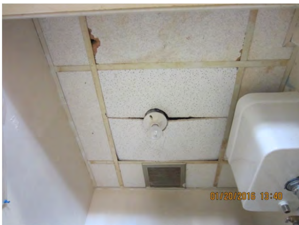
Photo 4.5.33 – Damaged ceiling tile in Janitor's Room
