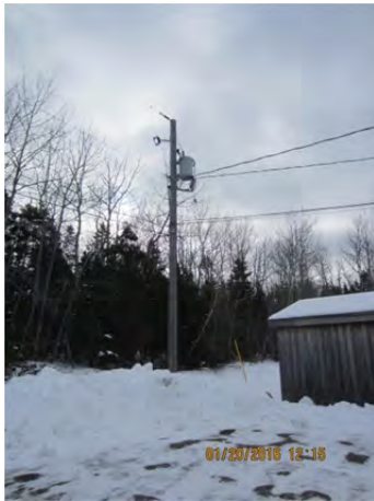
Photo 4.5.1 – 50 kVA single-phase pole mounted utility transformer
