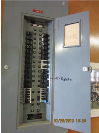
Photo 4.5.7 – Typical 100A, 120/240V, 1-phase, 3-wire Federal Pioneer distribution panel located in the school corridor
