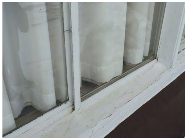
Photo 4.2.4 – Wood framed windows along the north face. Some paint peeling.
