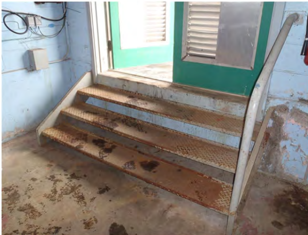
Photo 4.1.9 – Corroded stair into mechanical room
