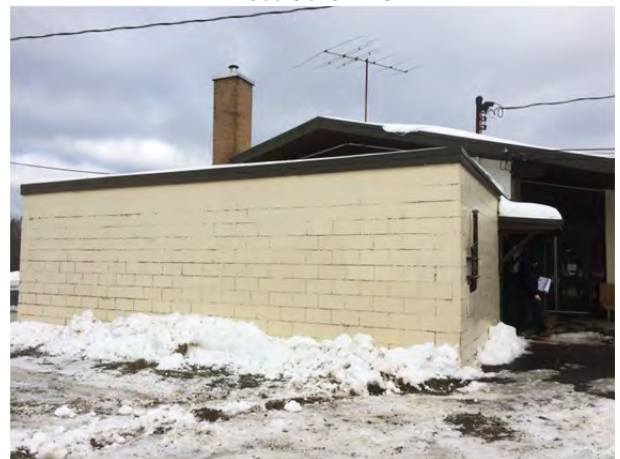
Photo 4.2.12 – East face of the boiler room. Painted joints in concrete block peeling
