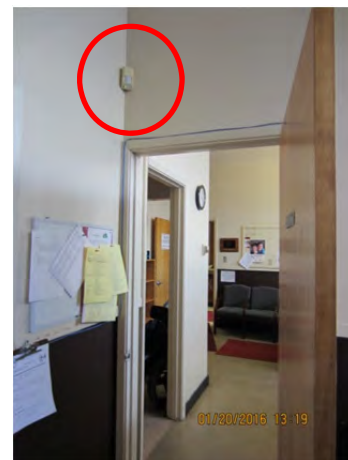
Photo 4.5.28 – Typical wall mounted motion sensor
