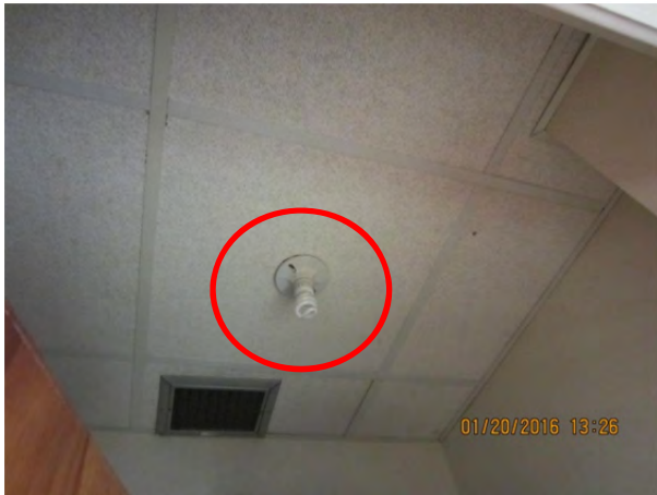
Photo 4.5.13 – Typical A19 luminaires in Janitor, storage and small washrooms
