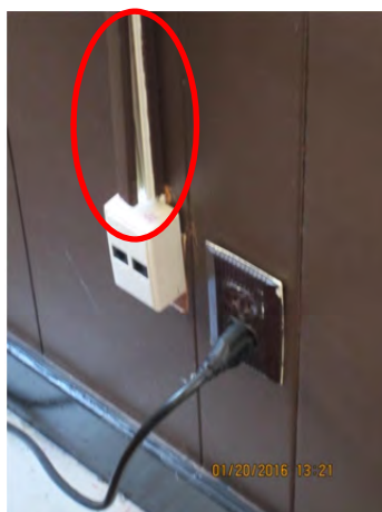
Photo 4.5.29 – Unsecured wire mold in Principal's office
