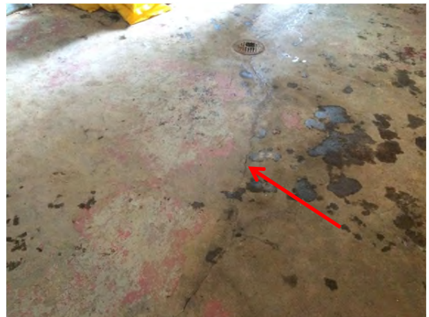
Photo 4.1.4 – Exposed grout and area of material loss. Southeast corner of mechanical room
