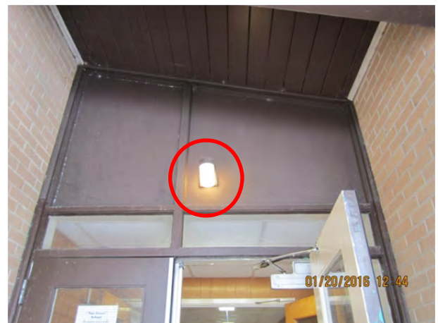
Photo 4.5.18 – Typical wall-mounted luminaires at the school entrances
