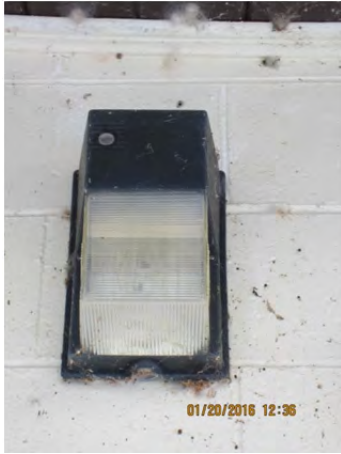
Photo 4.5.19 – Typical wall-mounted HID luminaires mounted on school perimeter
