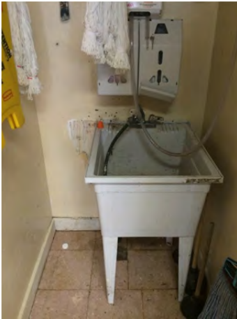
Photo 4.8.3 – Janitor Closet. Water damage to wall and floor.
