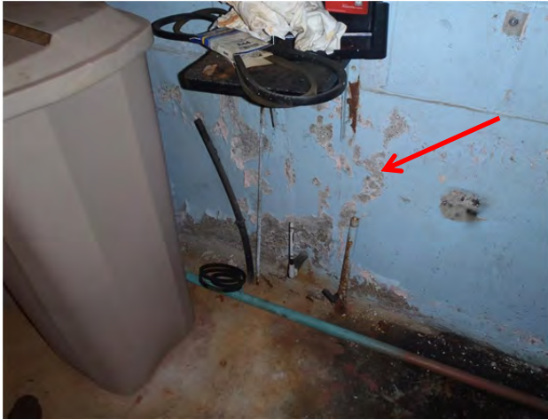
Photo 4.1.7 – Concrete spalling on interior of mechanical room foundation
