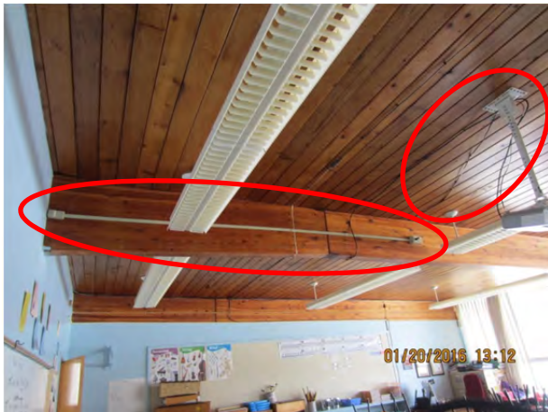
Photo 4.5.9 – Typical wiremold and wiring for ceiling suspended projectors
