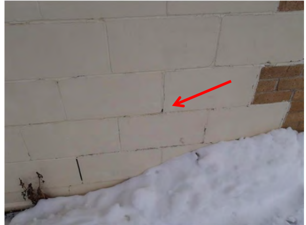
Photo 4.1.2 – Cracks and deteriorated mortar on northeast corner
