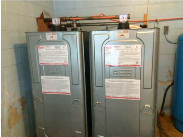
Photo 4.4.1 – Roth fuel storage tank for the building's heating system.
