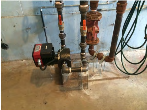
Photo 4.4.3 – Heating circulation pumps
