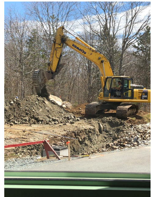
Breaking ground at Liverpool Regional High School's new skilled trade centre.
